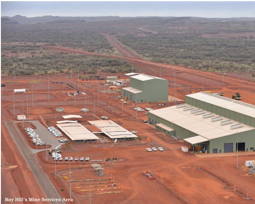
Roy Hill's Mine Services Area
