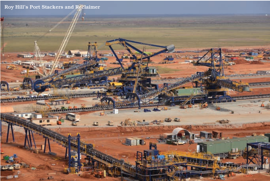
Aerial view of Roy Hill's Train Load Out Facility
